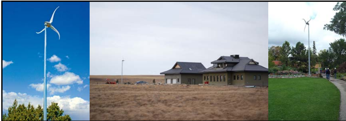
Figure 2: Typical micro-wind installations
