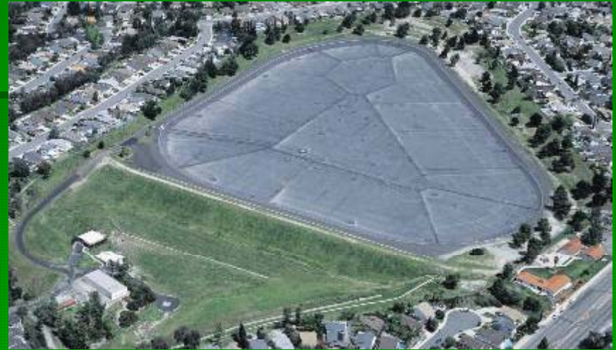
Large potable water floating cover El Toro CA
