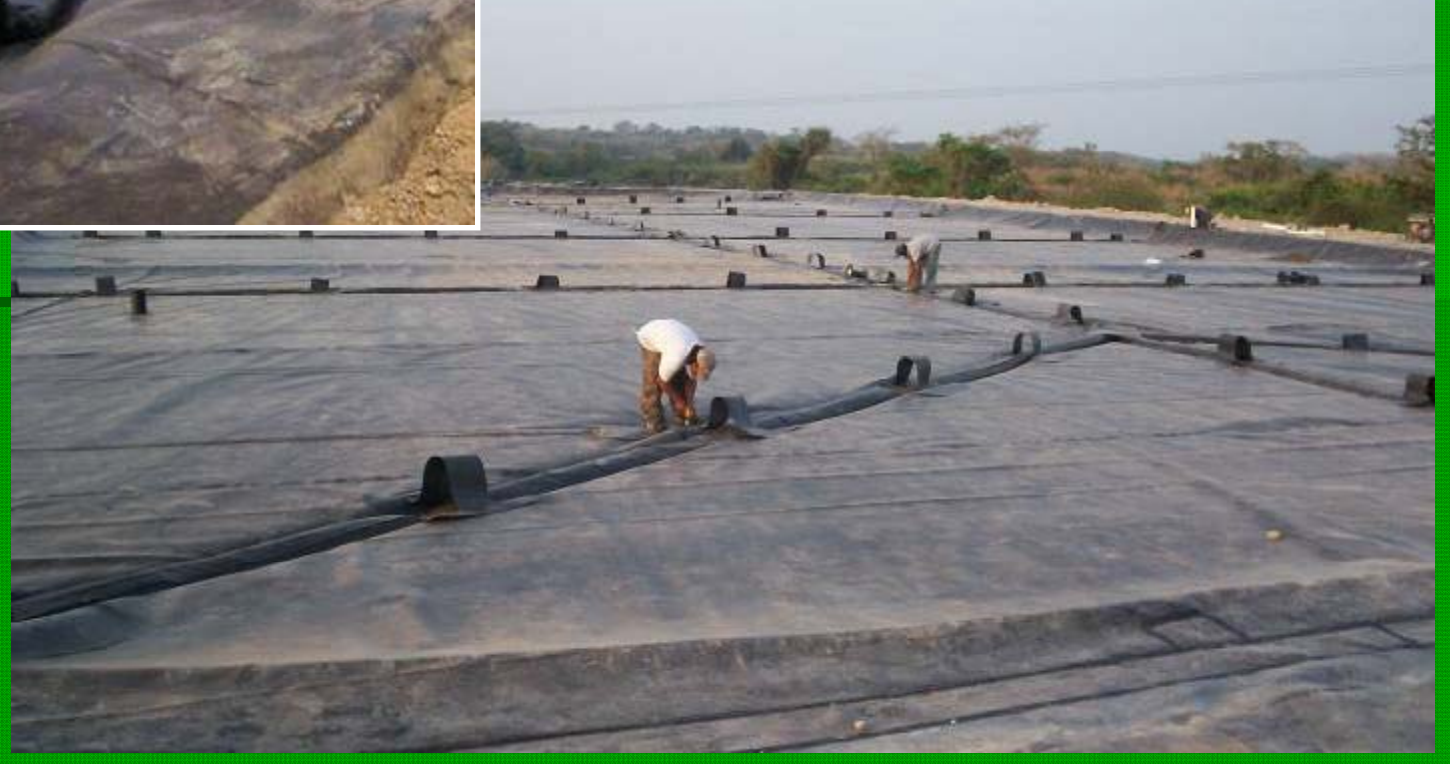
Secure cover weights with straps
